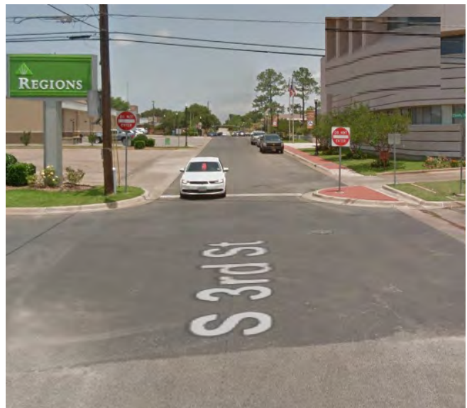
South 3rd street is an example of a two-way street conversion to a one-way street. The red brick bulb out and the Do Not Enter sign indicates to the driver about the conversion. Source: Google Street View
